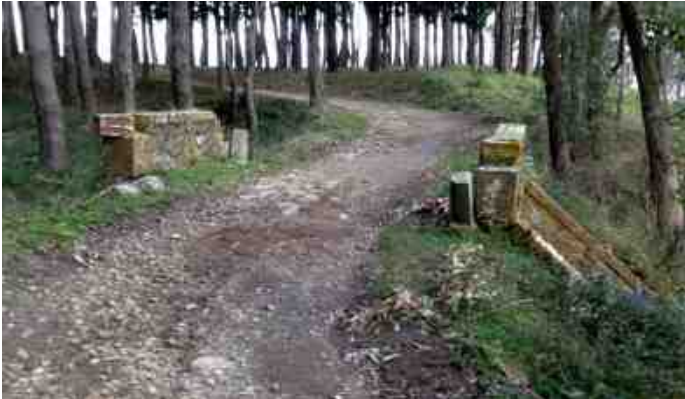
Fig. 2 - Underpass for the downflow of rainwater and stone post. Loc.: Campone Fort (North-Eastern Peloritani Mts.).
