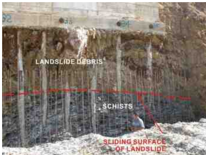
Fig. 7 - The cut of the slope foot
