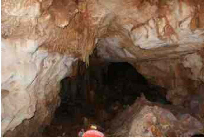
Fig. 4 – SE branch of the system, showing in the foreground breakdown deposits (see also the shape left by the rock failures on the cave ceiling).
