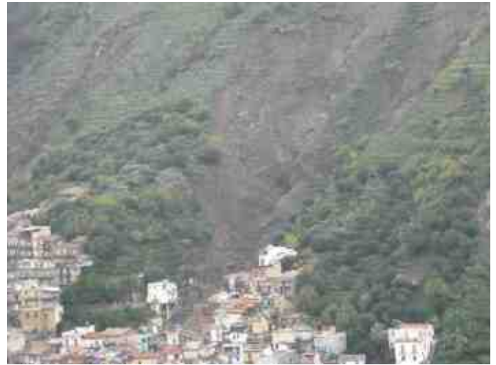
Fig. 2 – High erosion on the slope
