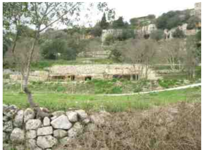
Fig. 1 – Consolidations Gymnasium stone walls in Cava d'Ispica and the result of the ecological restoration in 9 months.
