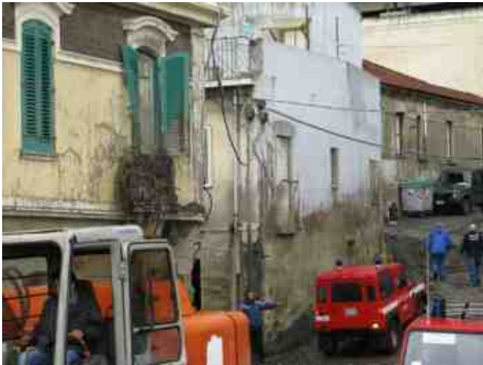
Fig. 1 – Damages in the Scaletta Zanclea area.
