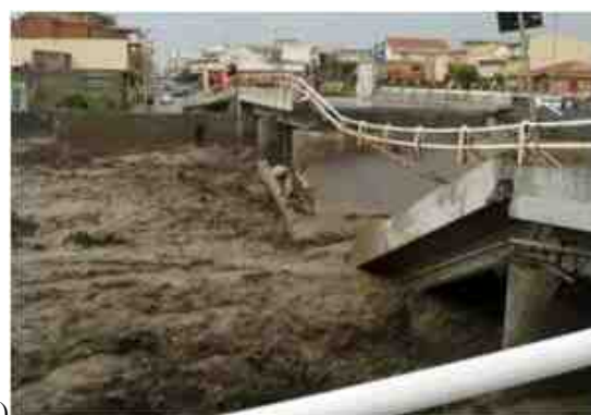
Fig 2 - Images of the alluvial events: a) heavy damages in the urbanized area of Giampileri during the alluvial event of 1 st October 2009; b) bridge collapsed in Barcellona Pozzo di Gotto town during the alluvial event of the November 2011.
