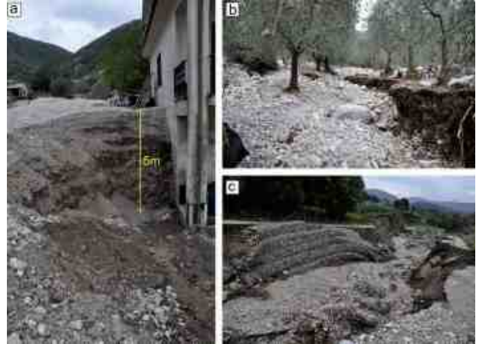
Fig. 2 – Alluvial deposit observed close to the wall of house facing upslope (a) and in the riverbed (b) of Maturra creek; c) the debris deposited in the riverbed of the Vadursi creek and observed damages to the gabion walls.
