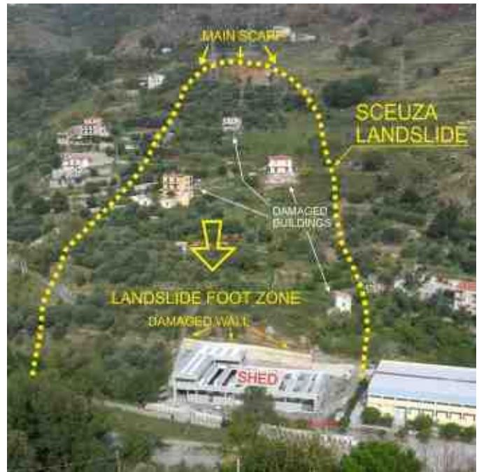
Fig. 1 – Landslide on the slope of Scèuza, (Cetraro, CS).
