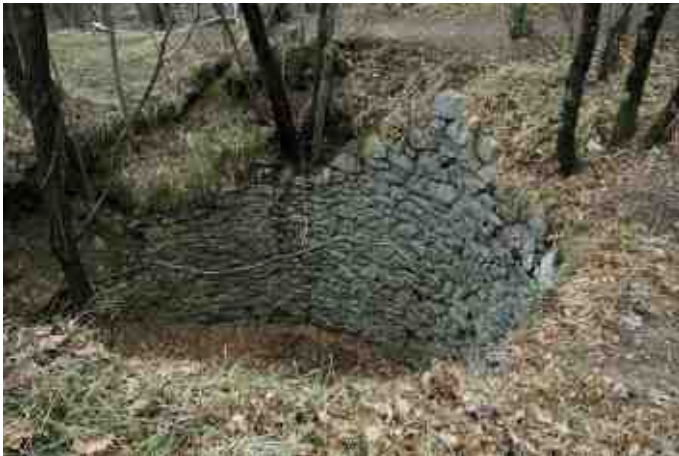
Fig. 3 – Remains of an ice-house, where the ice forming in Winter in the nearby ponds was deposited and conserved. The ice was sold in Summer before the development of modern refrigeration systems. Obtained from materials of colluvial origin, the man-made facility was made of limestone.
