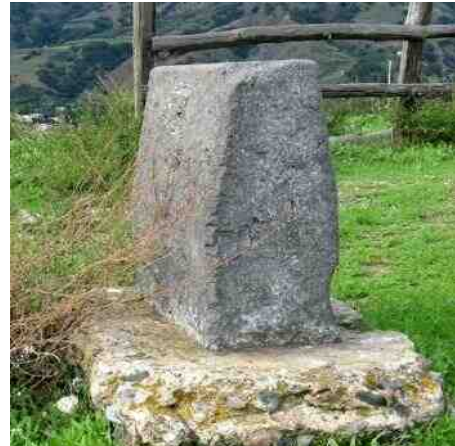
Fig. 4 - A milestone, indicating kilometric distances, made up of an Etna basalt block. Loc.: Cavalli Fort (North-Eastern Peloritani Mts.).
