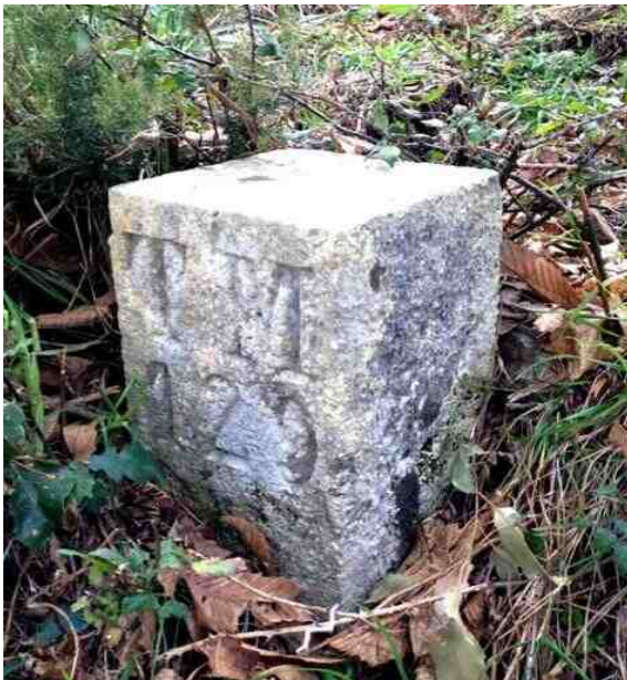
Fig. 3 - A milestone, indicating kilometric distances, made up of Aspromonte Unit late-Variscan pegmatite. Loc.: Military road between Puntal Ferraro Fort and Campone Fort (North-Eastern Peloritani Mts.).
