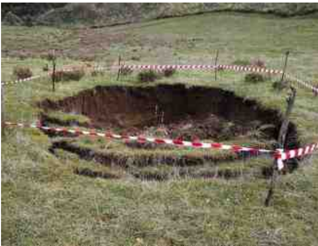
Fig. 2 – Geomorphologic evidence of the sinkholes #2 (top) and #4 (bottom).
