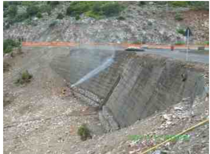
Fig.6 – Hydroseeding of reinforced soil
