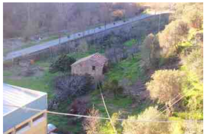
Fig. 9 - Ultra secular building partially built into the slope foot.
