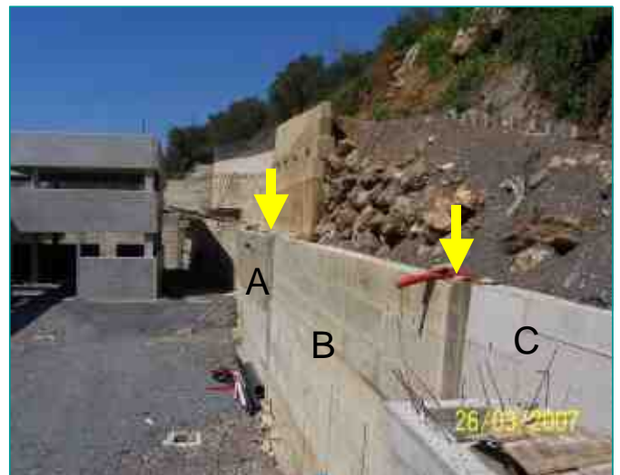
Fig. 5 - First displacements of the retaining walls
