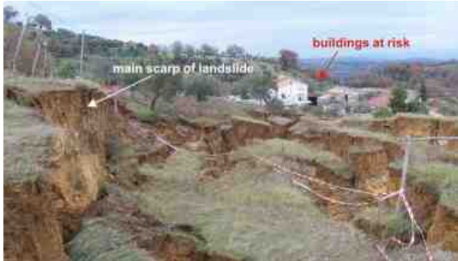
Fig. 2 – The landslide of Stragola (Montalto Uffugo) was being monitored by the A.M.A.Mi.R. system. Note the main scarp of the landslide and the buildings at risk.
