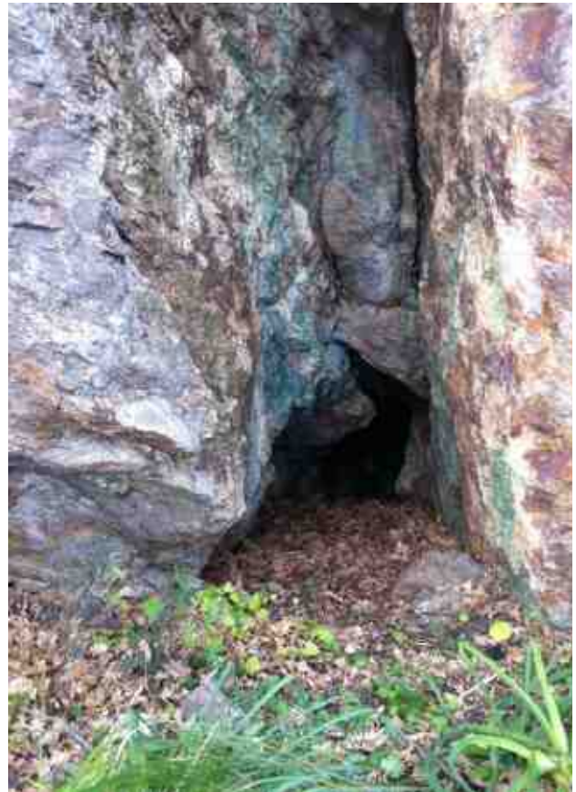
Fig. 3 – Entrance to a tunnel of the San Carlo mine, partially obstructed by debris.
